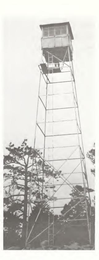
Figure 47. Promontory lookout, an Aermotor LS-40 with a 120 feet high tower, on Sitgreaves National Forest, Arizona. It was constructed in 1924 to replace the wooden tower in Figures 13 and 14. Photograph made by F. L. Kirby in 1934 (U. S. Forest Service photo 288837).
